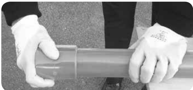
7. Wipe off excess cement from the outside of the joint.
