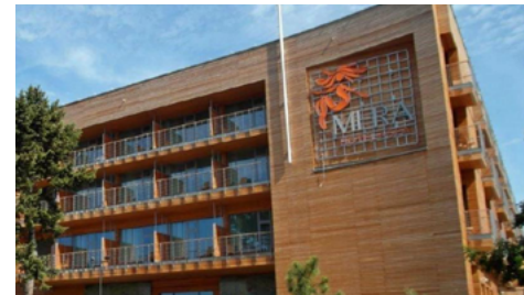
Mera Spa Hotel • 1700m 2 • 27 roof outlets
