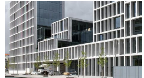
Bestseller Offices • 4600m 2 • 50 roof outlets
